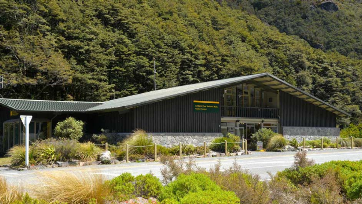
DOC Head Quarters (Visitors Centre) ICP for major events
