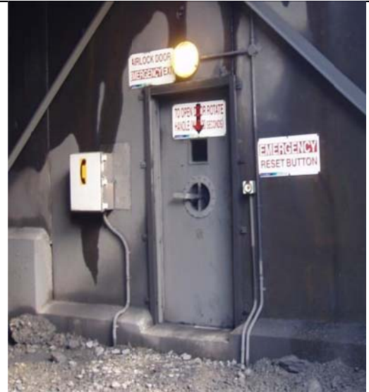
Picture 2: Airlock room inside tunnel entrance
