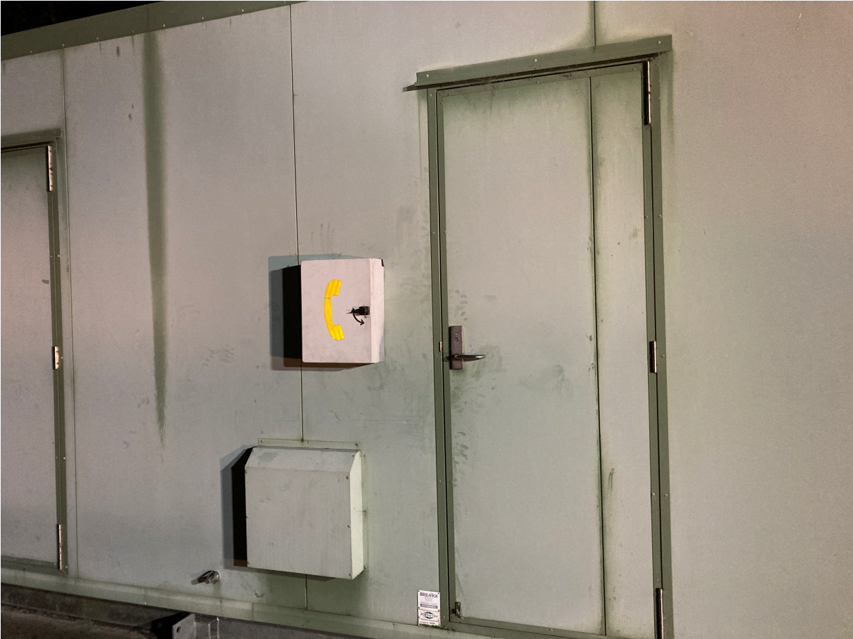
This radio is in a steel box on the front the point of supply building.
