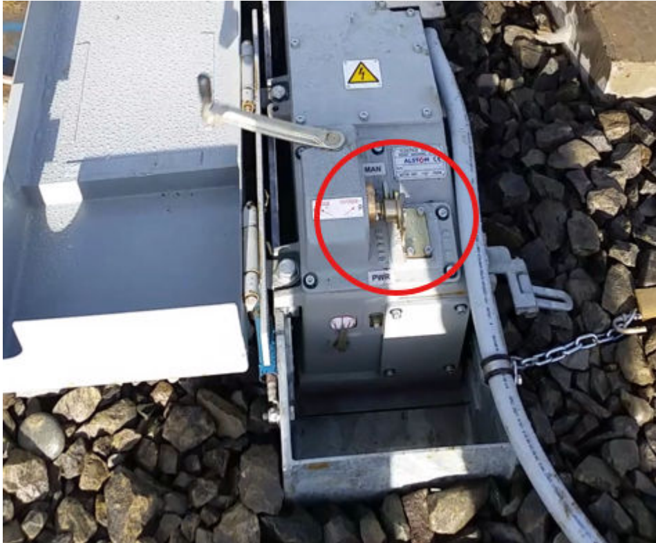
CTS2 Points Machine Isolator Ring
