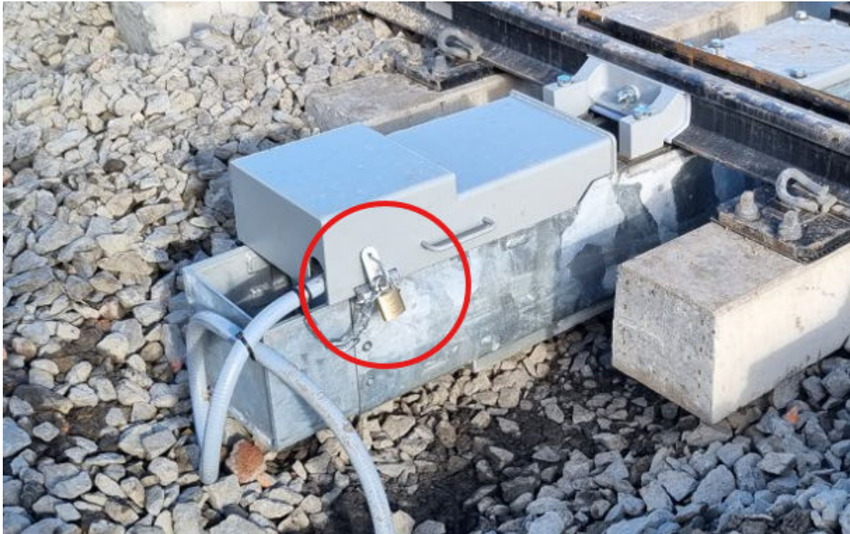
CTS2 Points Machine with locked cover
