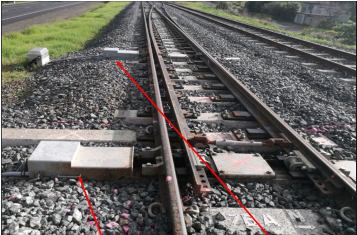
Left Arrow - the 'a' Points Machine
