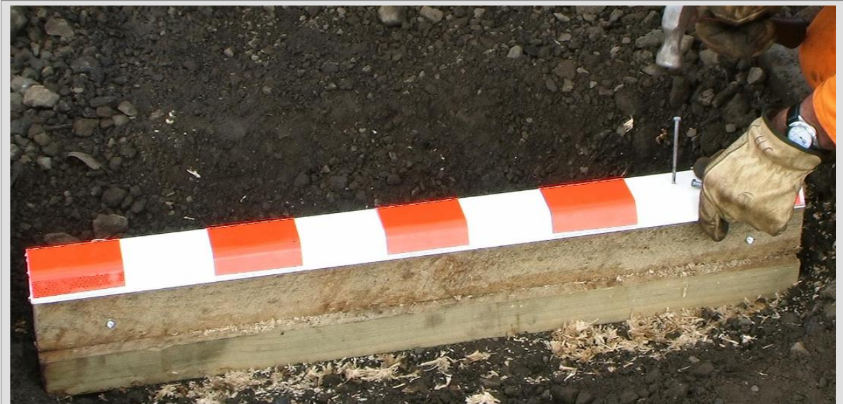
Fouling Point Marker
