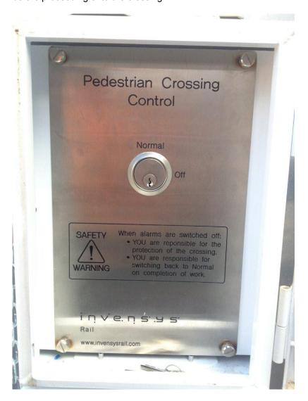
When manually cancelled or cancelled automatically after the train has passed over the crossing, if the train remains in the track circuit controlled area for a prolonged period the alarms may reactivate and should be manually re-cancelled. Manual controls must not be used to cancel alarms operating due to fault conditions.
