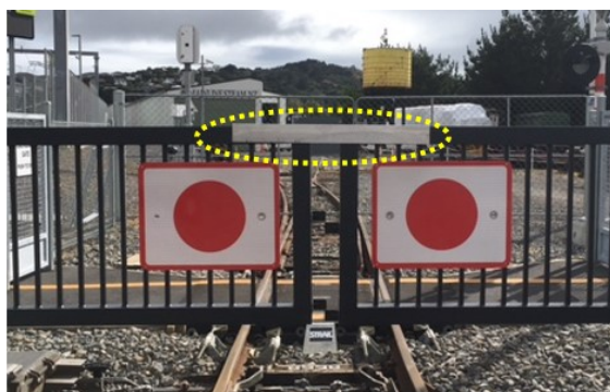
Gates locked by horizontal bar (L), Gates unlocked (R)
