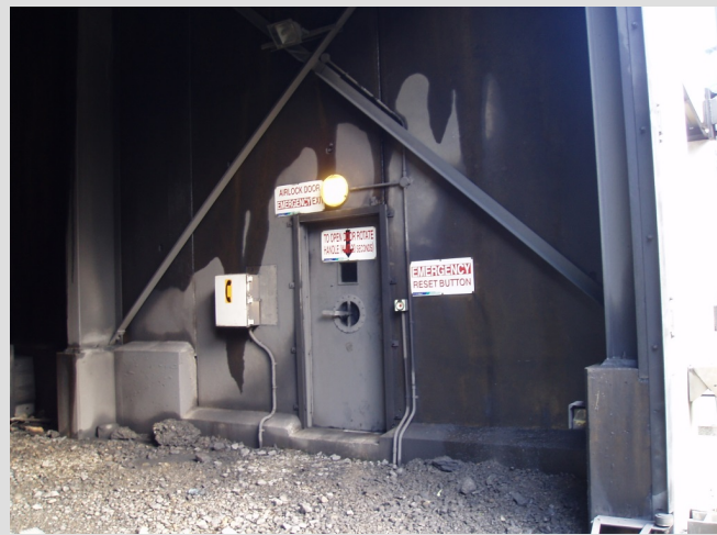
Picture 2: Airlock room inside tunnel entrance
