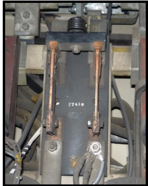
Figure 22: Knife Switch – Closed
