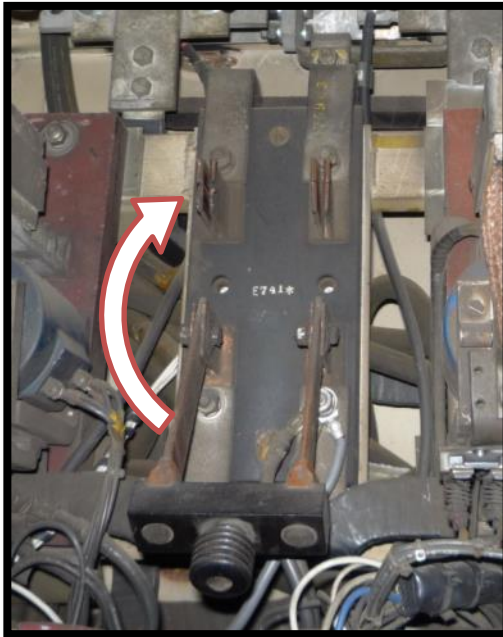
Figure 21: Knife Switch – Open
