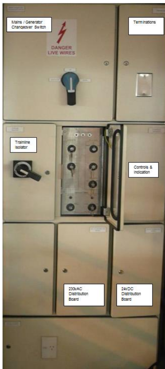
Figure 1: AKV switchboard
