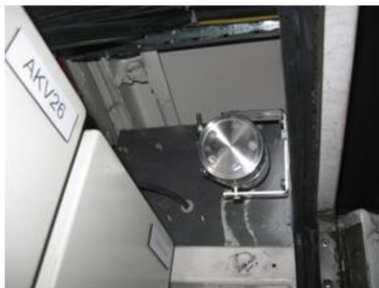
Figure 19: STAT X 100T aerosol generator.
